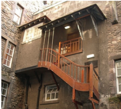
PRESENT: Exterior view of courtyard facade
