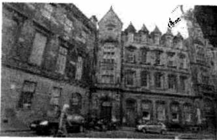
India Buildings, Victoria Street
